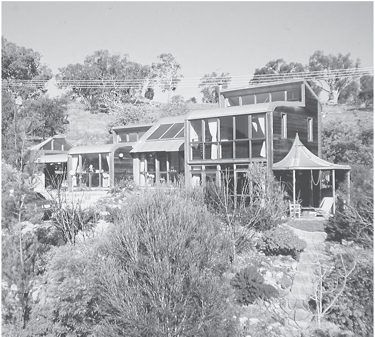
The 153 square metre home in Canberra requires no cooling and virtually no heating.
