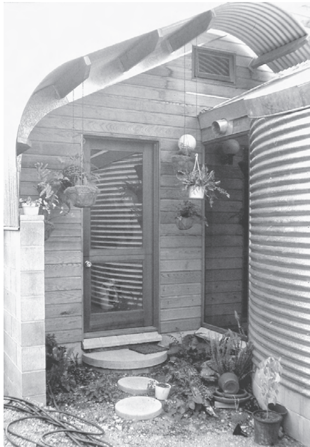
The east-facing 'back' door and south-facing shower recess window (double glazed reflective) with their fernery getting started.
